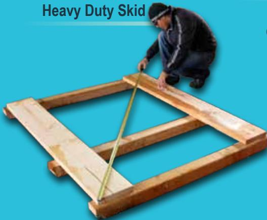
A counter sunk carriage bolt at four corners secures a **Heavy Duty deck** to each skid...
